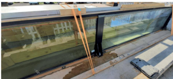
ABOVE: The glass panels are being installed as part of the Bewdley Left Bank Flood Risk Management Scheme.
