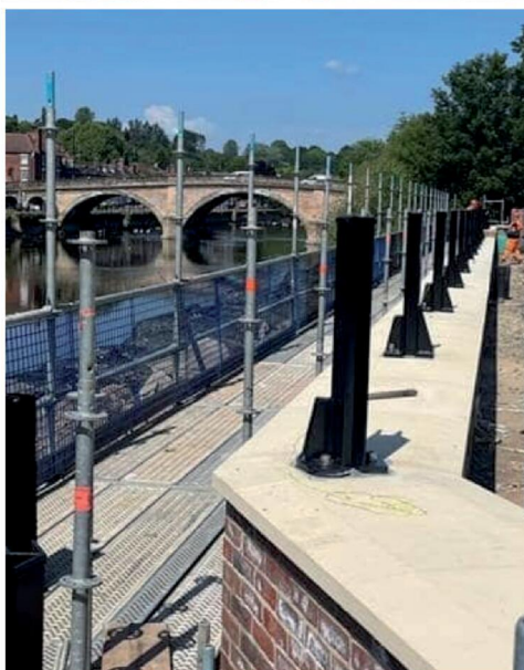
ABOVE: The glass panels are being installed as part of the Bewdley Left Bank Flood Risk Management Scheme.
