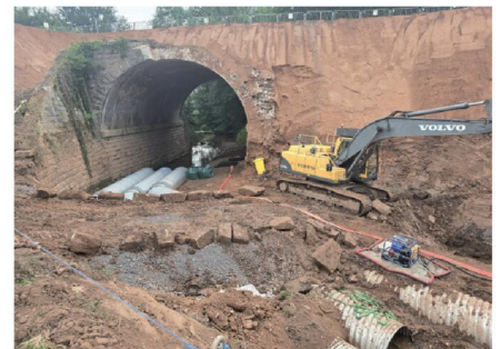
The contractor's workers covering the culverted watercourse. Picture by Antony Bartlam. s
